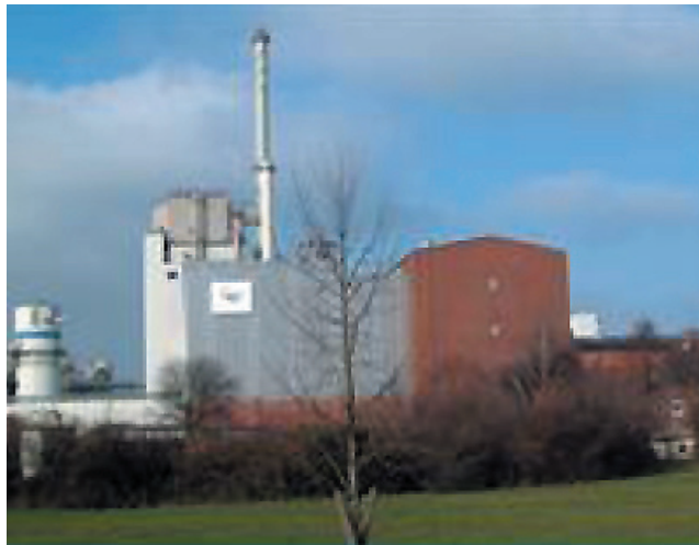
Pfeifer & Langen — packing centre and warehouse
